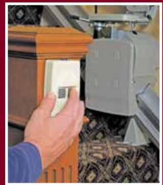
The two wireless call/send controls make installation simple and clean with no wires running along the wall.
